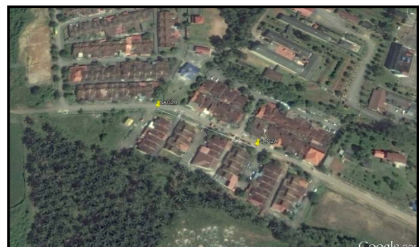
Fig. 8: The location and alignment of line SAG2 which is located along Jalan Kelemak Jaya
